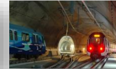
Dudullu Bostancı Metro Project
