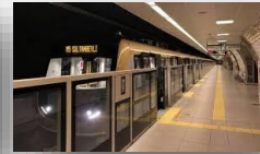
2 nd Phase of Çekmeköy Sancaktepe Sultanbeyli Metro Project
