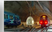
Dudullu Bostancı Metro Project
